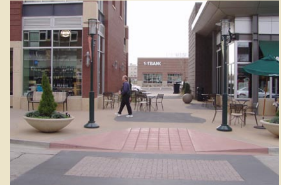
Use of textured or colored pavement for crosswalks increases pedestrian safety.
