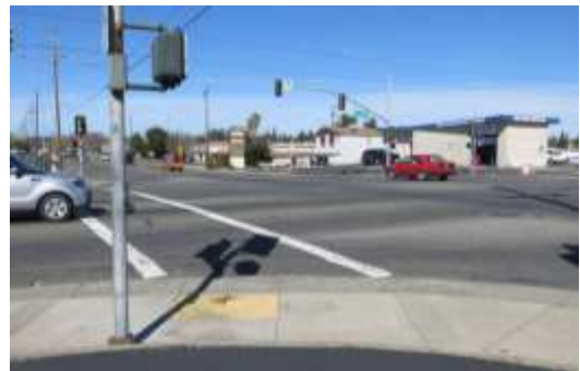
Intersection condition at Greenback Lane and Main Avenue.
