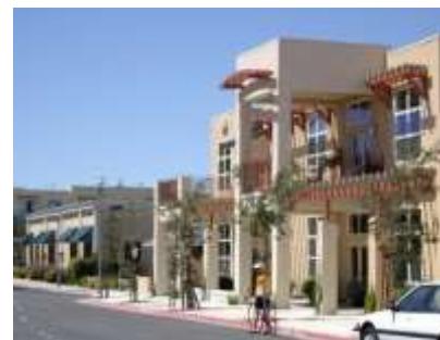
Buildings should have a clearly defined entry on M Street. Vertical elements, awnings, and overhangs can help to enhance entries.
