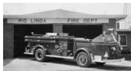
Rio Linda Fire Station, with partial stucco exterior and modified windows and door
