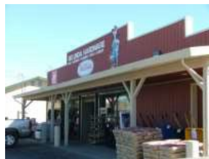
A typical commercial building, with flat roof and false front, wood siding, and an awning
