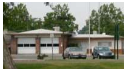
Rio Linda Fire Station showing original brickwork
