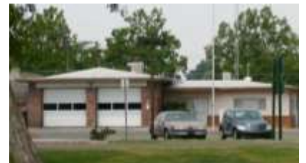
Rio Linda Fire Station showing original brickwork
