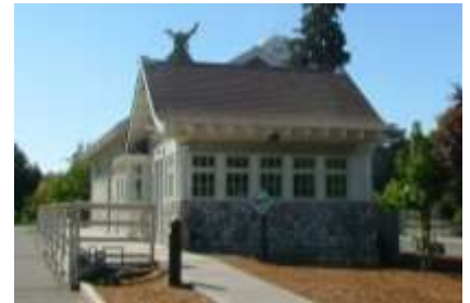
The Chamber of Commerce, housed in the reconstructed Train Depot, is an effective example of new construction that uses durable materials and high-quality construction that complements, but does not mimic materials found on other buildings in the Village Center.
