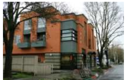
Buildings taller than two stories should be articulated to appear less massive.
