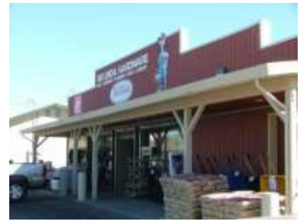
A typical commercial building, with flat roof and false front, wood siding, and an awning
