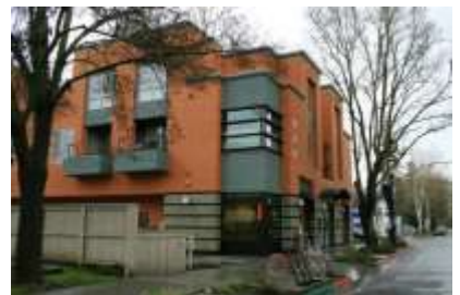
Buildings taller than two stories should be articulated to appear less massive.
