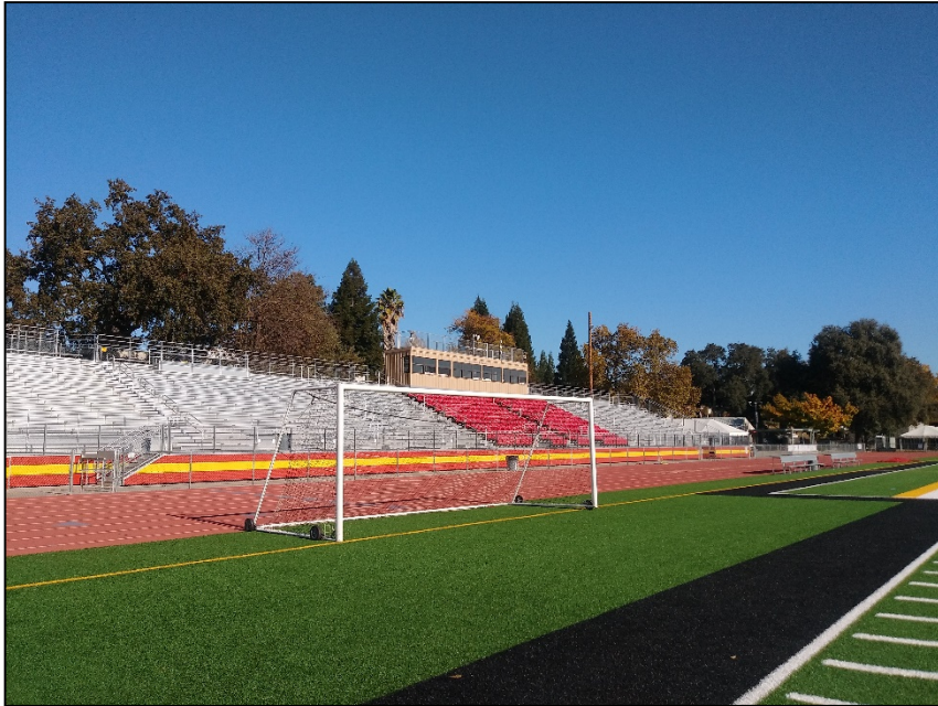
View from football field, looking northeast
