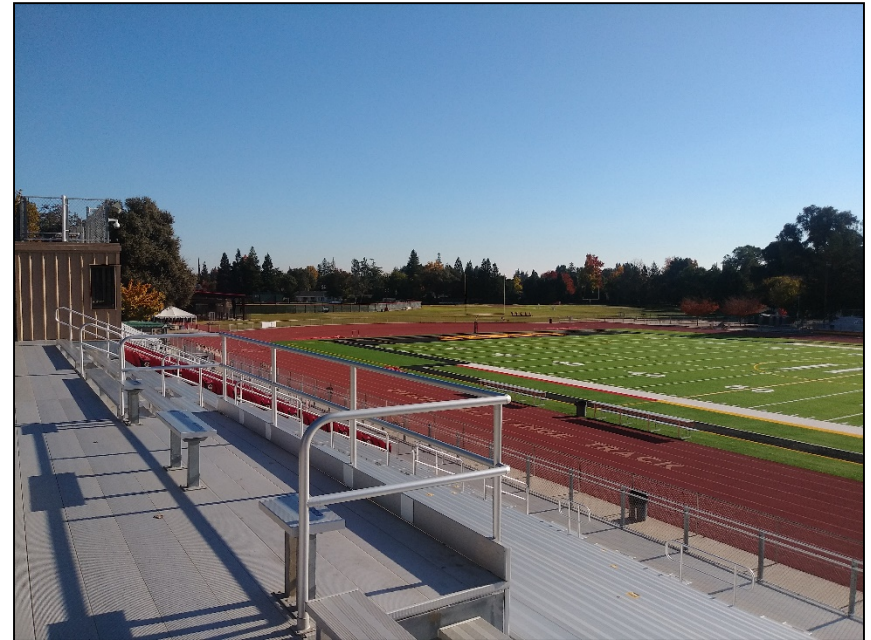
North side of stadium, looking southeast
